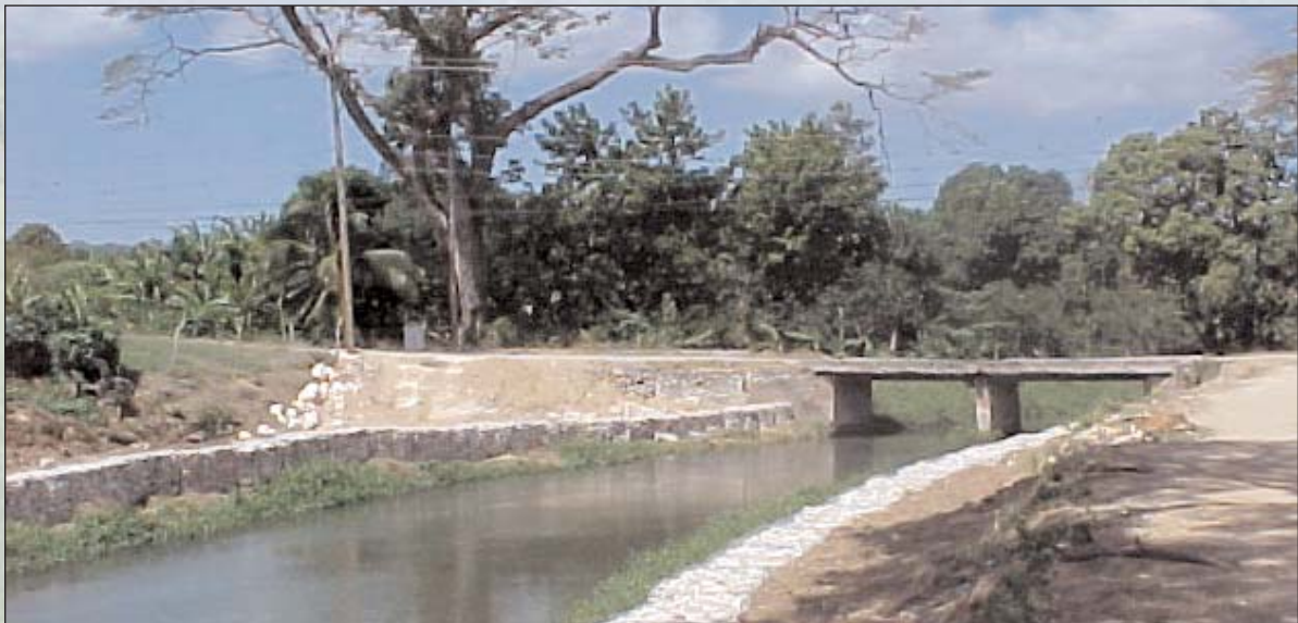
Gabion protection works on the Rio Cobre Main Canal completed under the IDB Flood Damage Rehabilitation Programme
