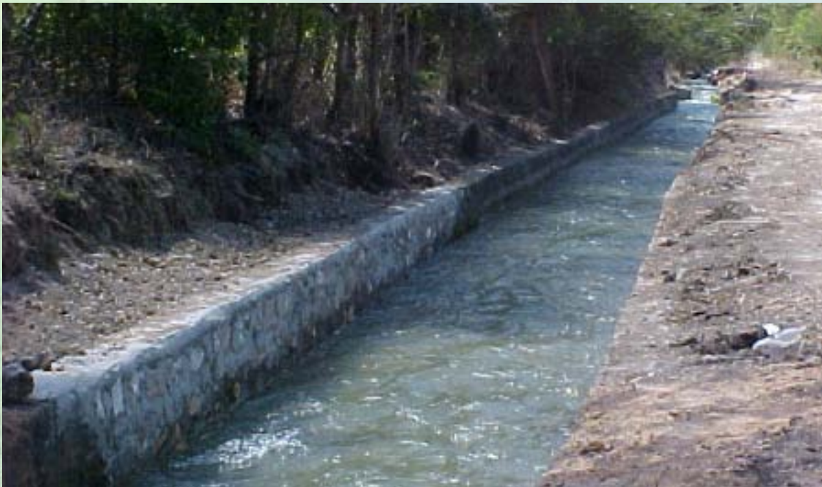
Finished stone masonry repairs under IDB Flood Rehabilitation Programme
