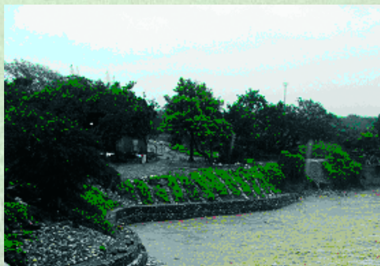
The completed gabion works at Rio Cobre, protecting the river bank and NIC works.
