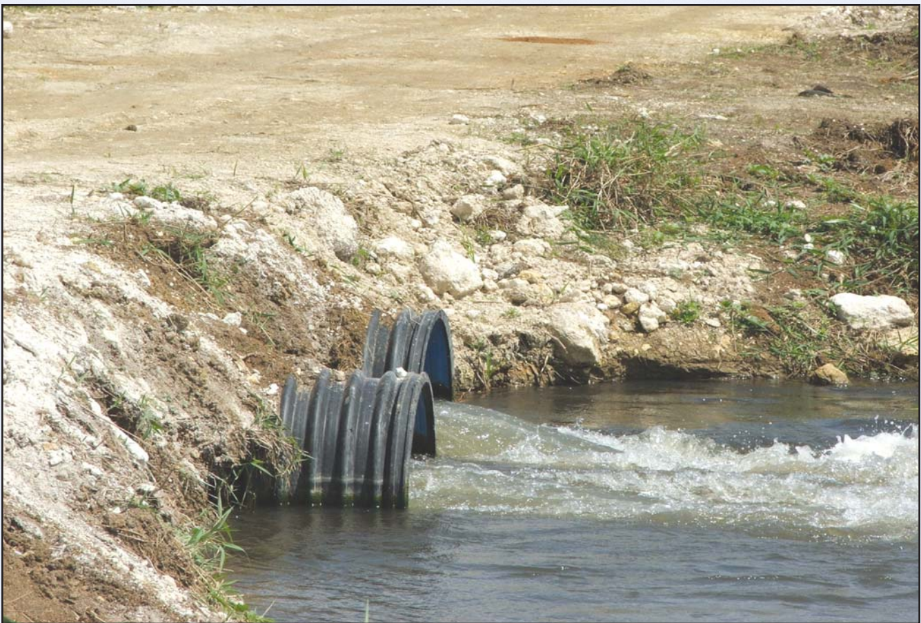
Fig 4: Culvert installed in the Drainage Area, St. Elizabeth
