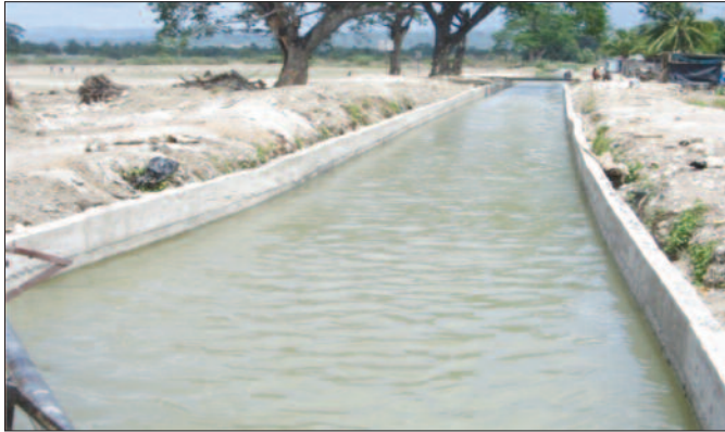
Re-lining of canal at Tawes Pen
