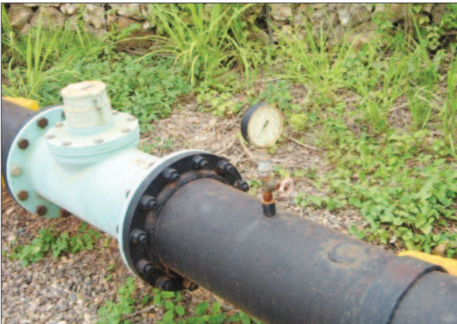
Installation of bulk flow meter in Hounslow
