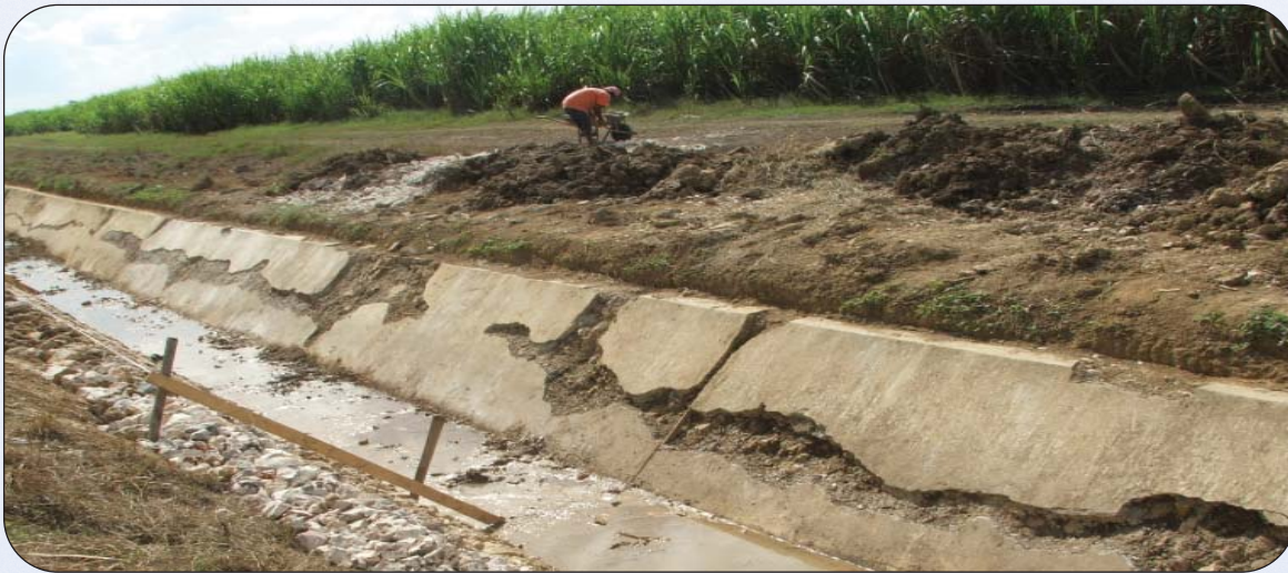
Repair to side of the Main Canal in Mid-Clarendon
