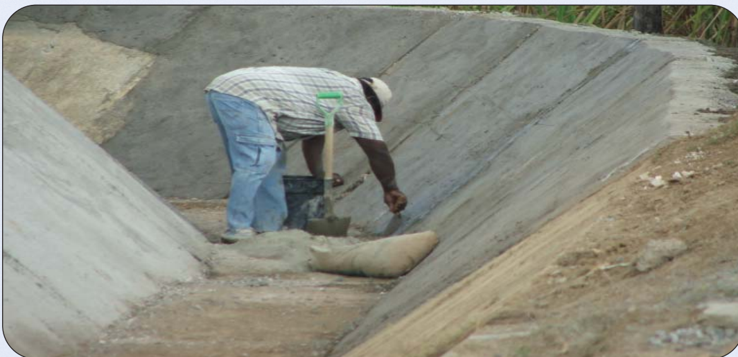
Canal lining of a section of the Main Canal, Mid-Clarendon
