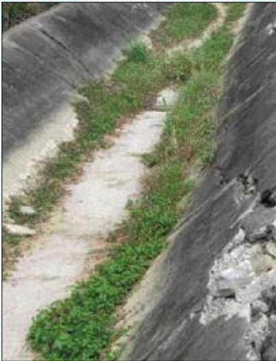
Deteriorated section of Old Milk River Canal stone packed trapezoidal canal
