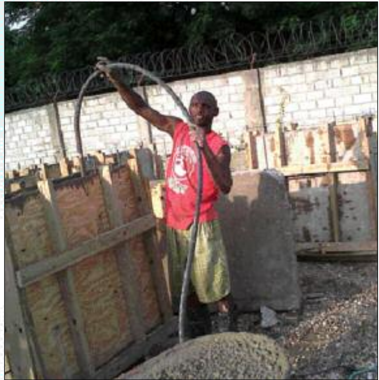
Pre-fabrication of rectangular walls section
