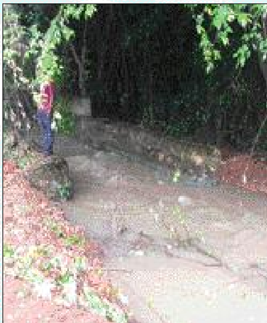
Section of the Old Harbour Main Canal in Innswood showing earth backfill to stabilize eroded bank
