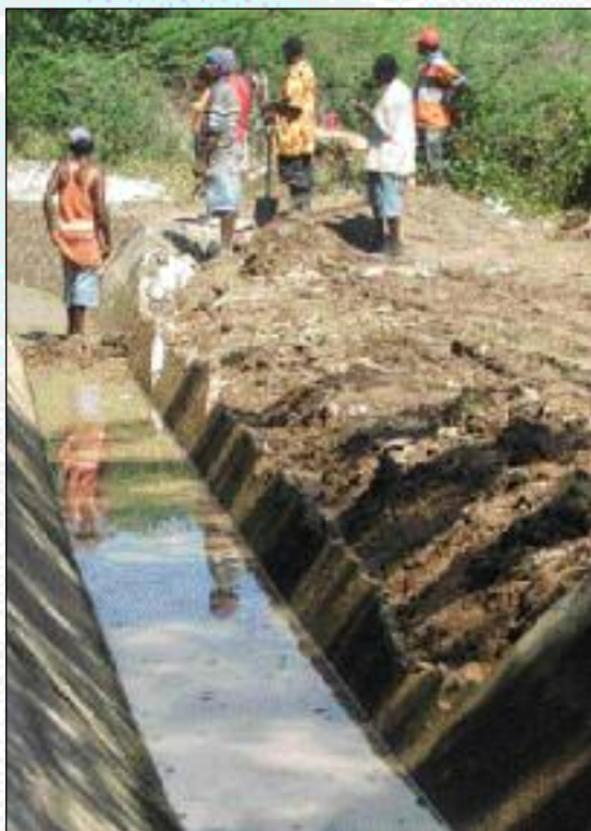
St. Dorothy Main Canal with damaged wall section removed
