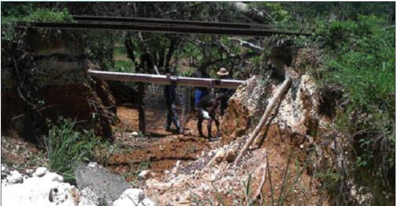
Seven Rivers pipeline repaired after being damaged by heavy rainfall and erosion
