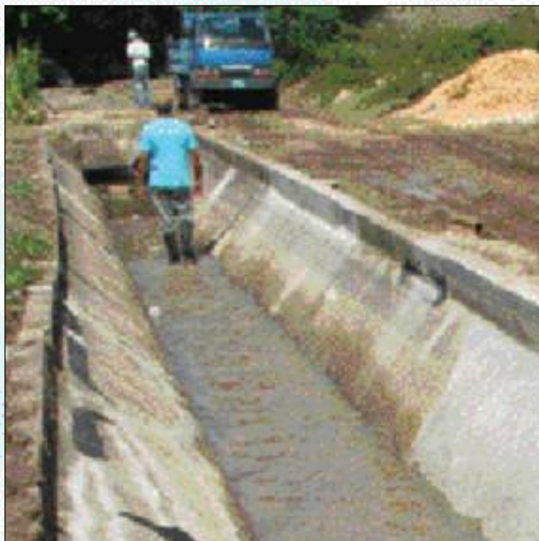
St. Dorothy Main Canal with damaged wall section repaired with concrete (approximately 600 ft of canal was repaired)
