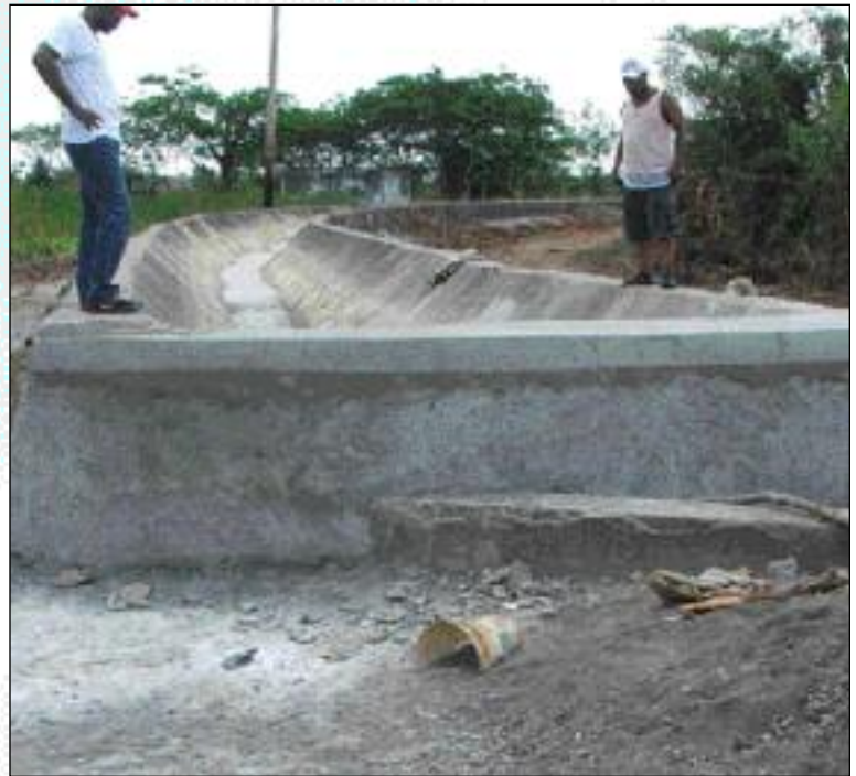
Approximately 1 mile of repairs to Old Milk River Canal wall and invert
