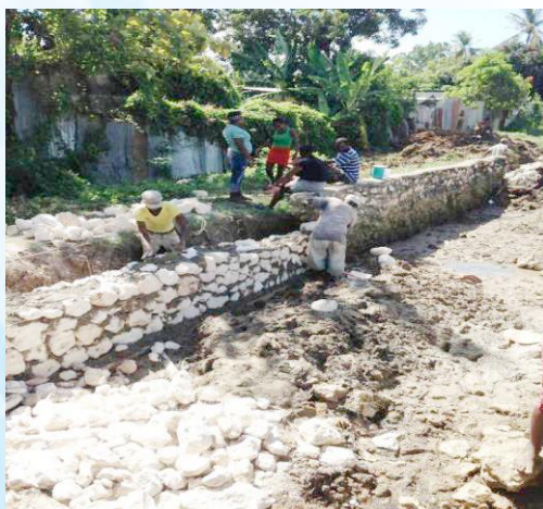
Old Harbour Branch Canal - Reconstruction of Stone Masonry Wall
