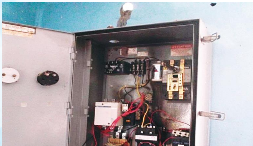
Motor Control Panel damaged by vandals
