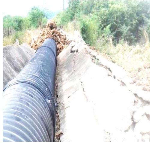
Old Milk River – Repair Using Pipes
