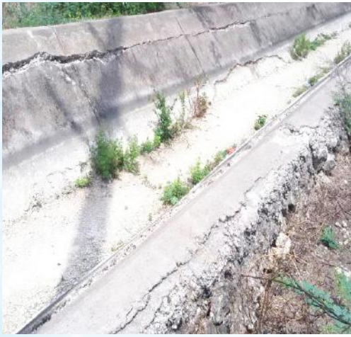
Old Milk River Canal – Cracked Sections
