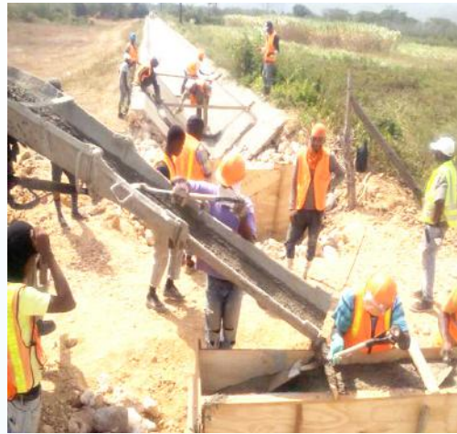
Old Milk River – Construction of Reinforcement Inner Lining
