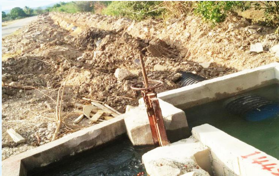
Rhymesbury Line 39 - Works advanced to complete HDPE pipe installation terminating in distribution chamber
