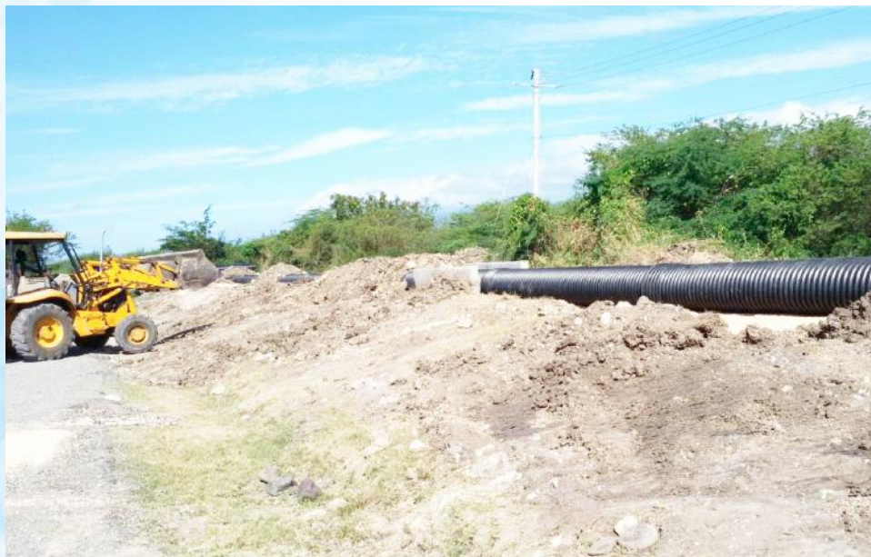
Rhymesbury Line 39 - New Reinforced HDPE Pipes being installed
