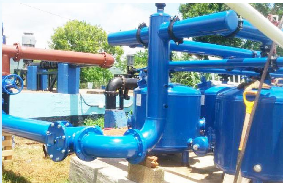
Gravel Filtration System Installed at Ebony Park
