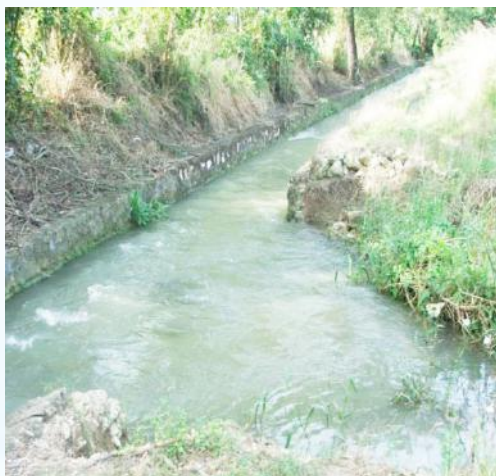
West Main Canal – Broken Sections
