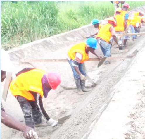
Old Milk River – Construction of Reinforcement Inner Lining
