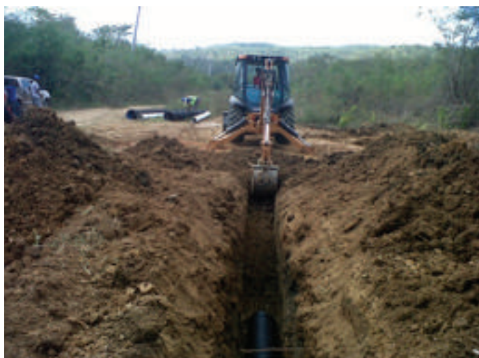
Pipe Trench Excavation at Spring Plain.
