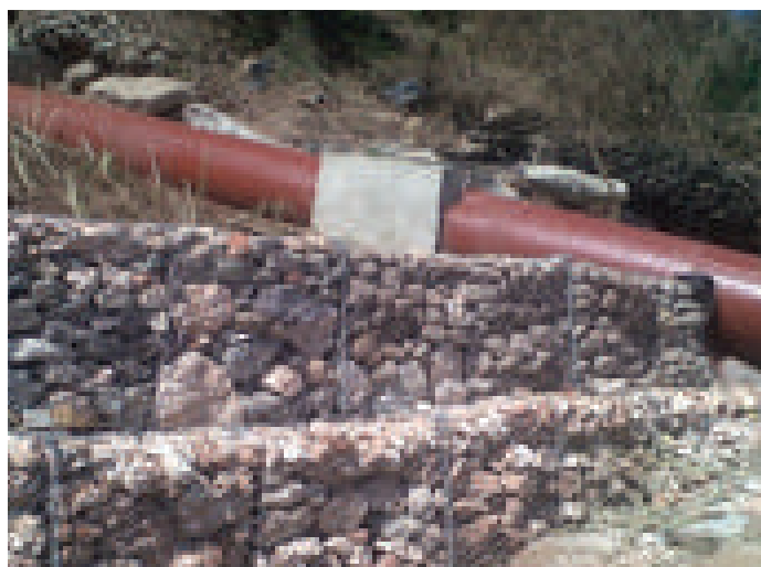
Canal Siphon Pipeline Crossing the Rio Cobre River.
