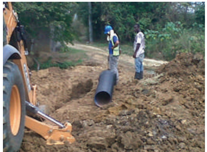
Excavating to Install River Crossing at Ebony Park.
