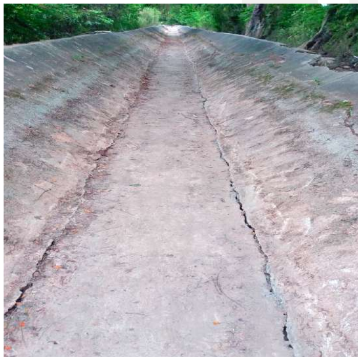
Figure #1: Canal bottom with cracks before rehabilitation work
