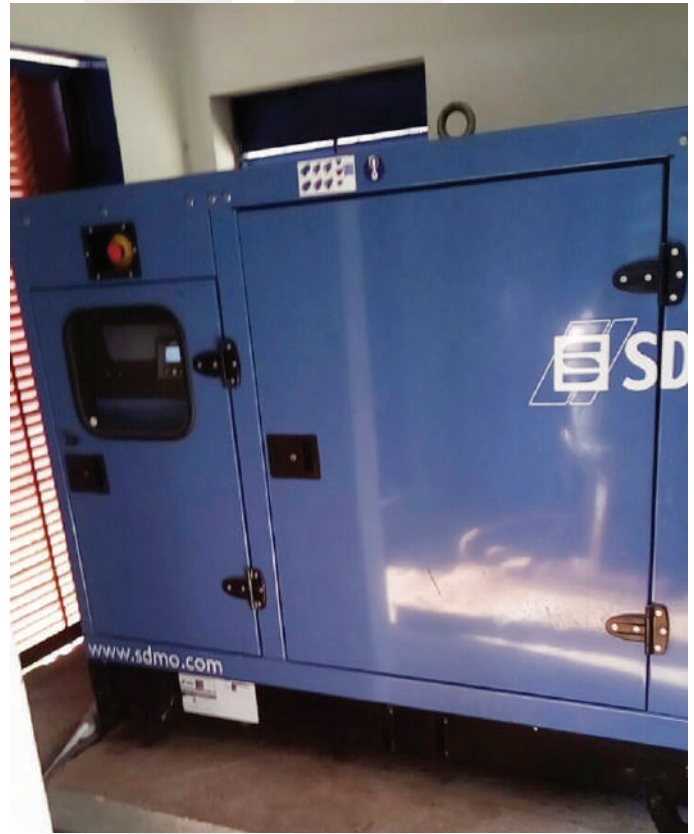
Figure#8: Standby generator installed at Cookson #4 pumping station
