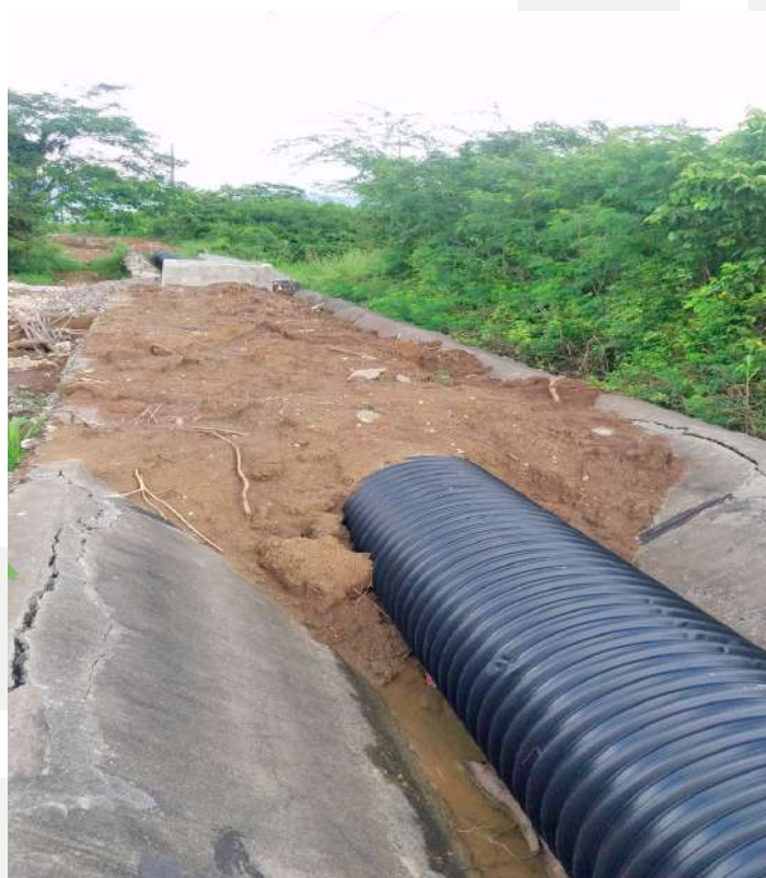
Figure # 2: showing Phase 4 of the project involved the installation of HDPE pipe to replace leaking canal
