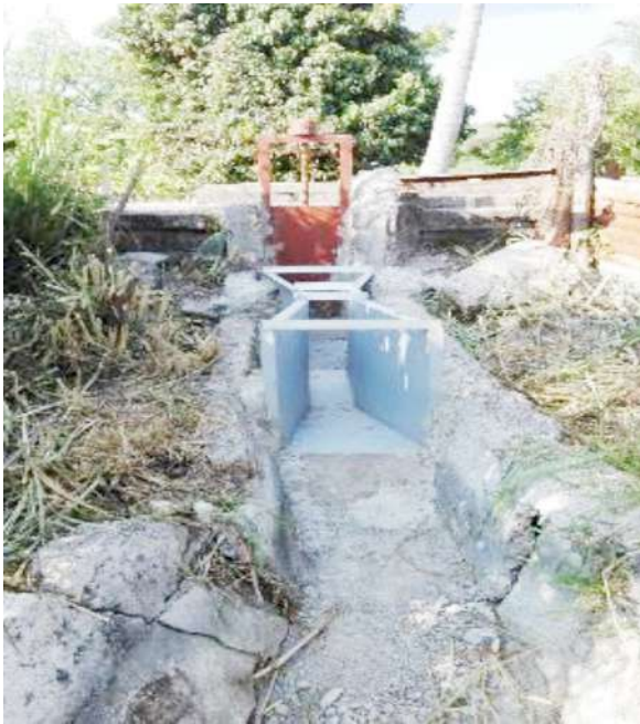
Figure#13: Sluice gate and parshall flume (measuring device foreground) at customer service point
