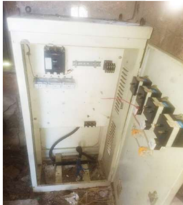
Figure #14: Thieves gutted a motor control centre.
