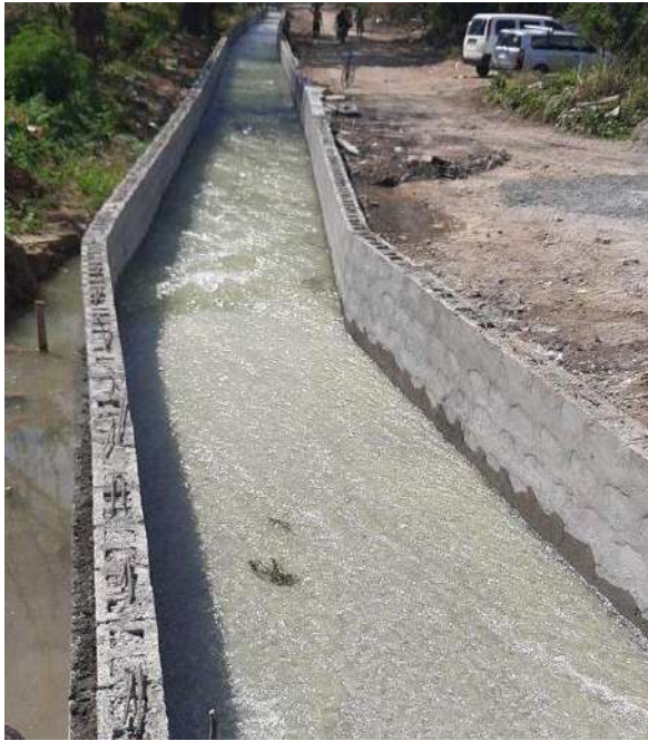
Upper Old Harbour canal restoration.
