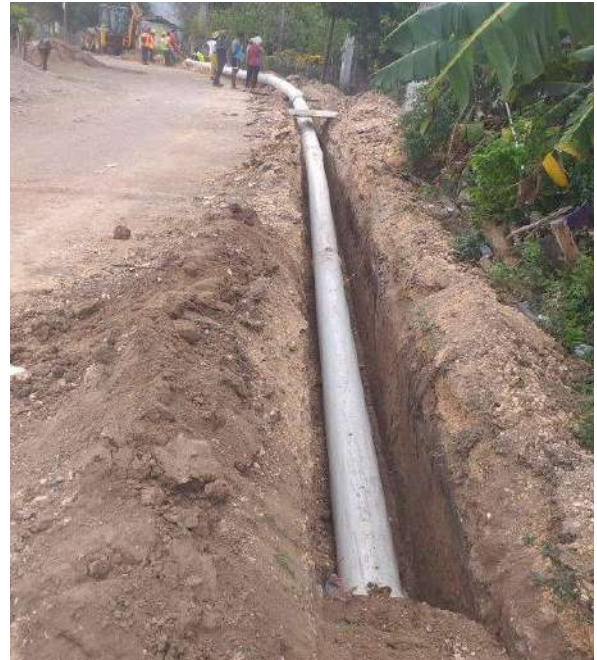
Upper Rhymesbury pipeline replacement project.
