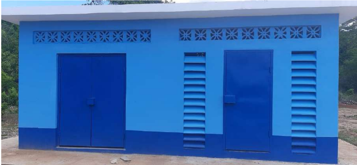
Thetford pumping station after renovation.
