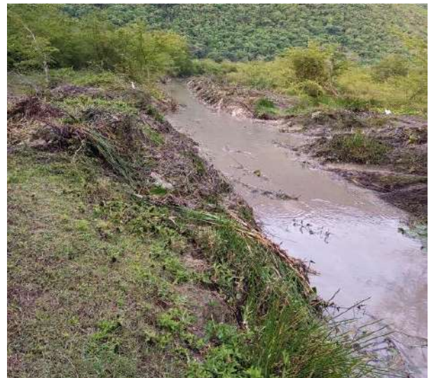
Mitcham canal after being mechanically cleaned.
