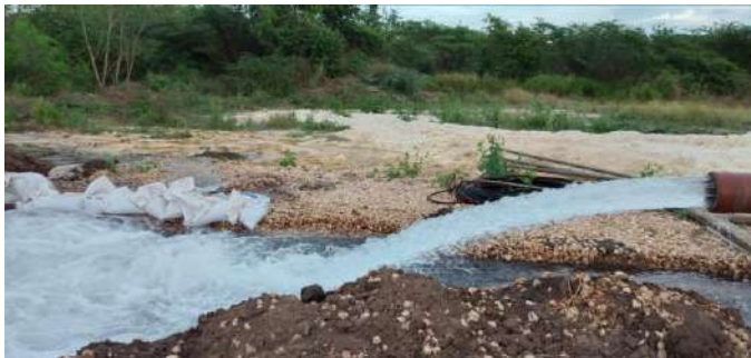
Yield testing of the well - Windsor Lodge 8R Well (SPAD)
