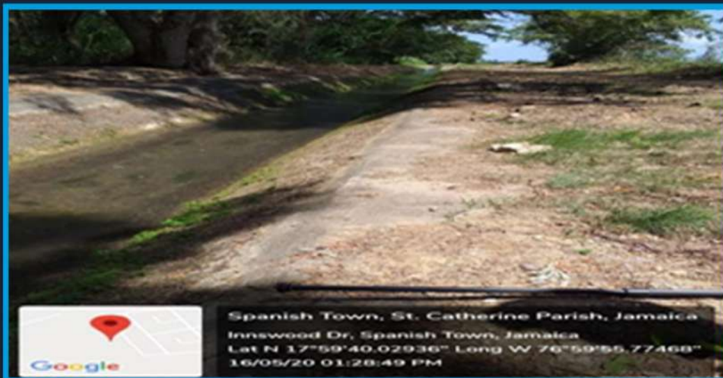
Section of the Hartlands Canal to be rehabilitated under SPAD Project
