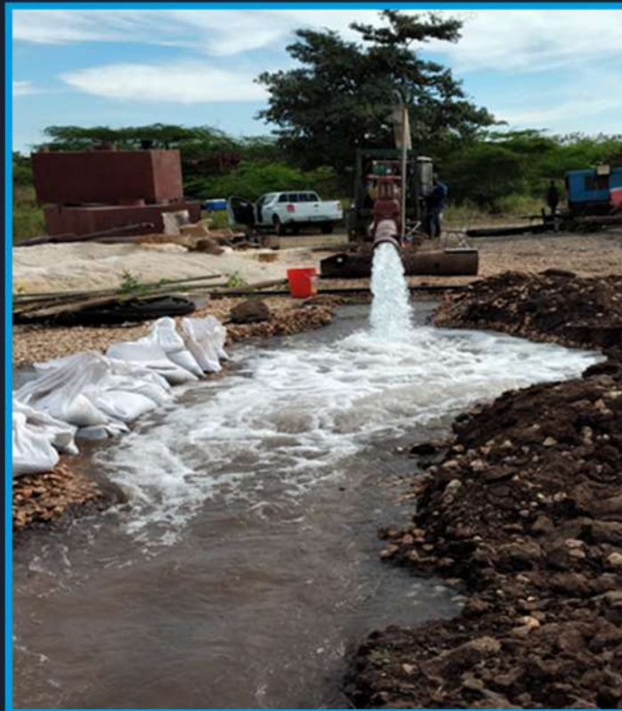
Drilling of wells, part of Irrigation Infrastructure Development Parnassus, Clarendon (SPAD)
