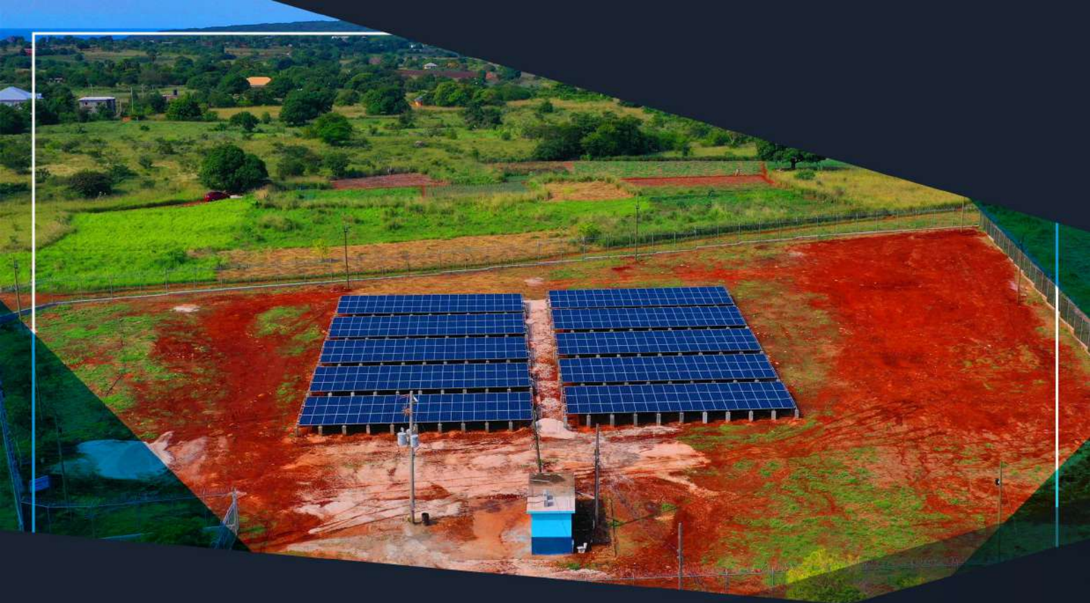
Beacon Little Park F3 pump station with 200 kW Solar PV system
