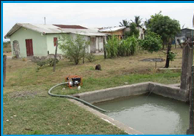
Water being stolen from the canal system
