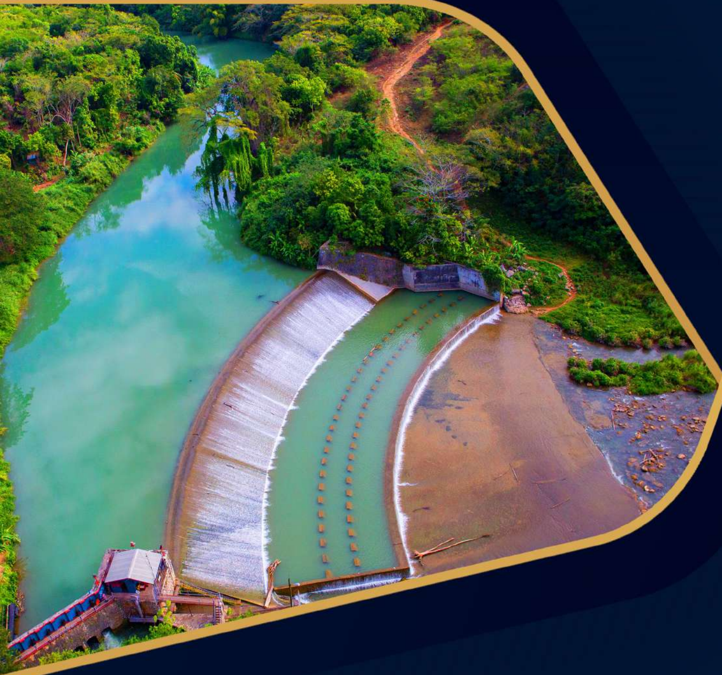
THE RIO COBRE DAM
