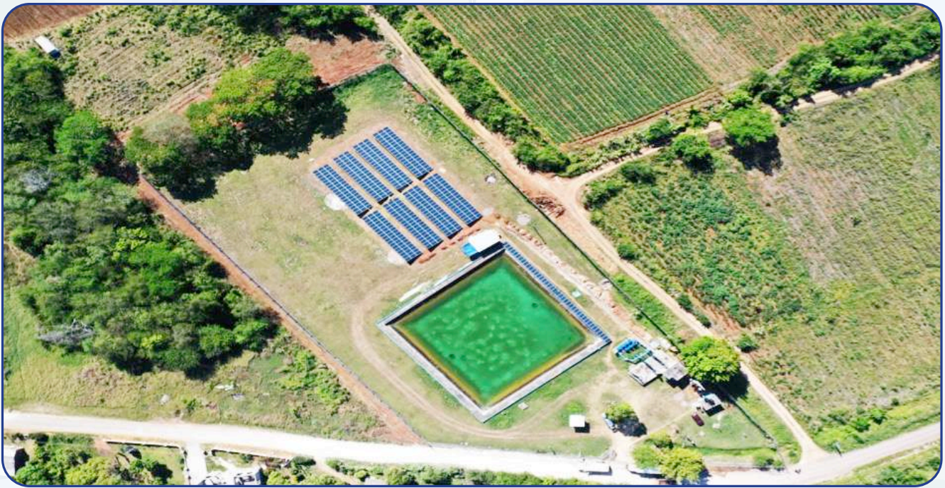
120kW Solar Retrofit of the Ebony Park Pump Station in Clarendon
