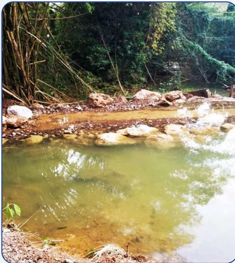
YS River Canal Diversion
