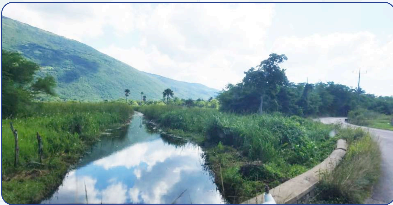
“Pass Water” in the parish of St. Elizabeth after manual cleaning
