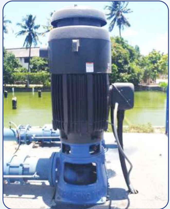
Pump Installation at Lane Pump Station and Premium Efficiency Motor Installed at Innswood Pump Station
