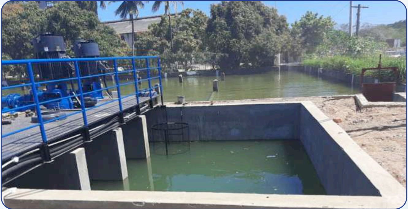
Completed Innswood relift sump and reservoir
