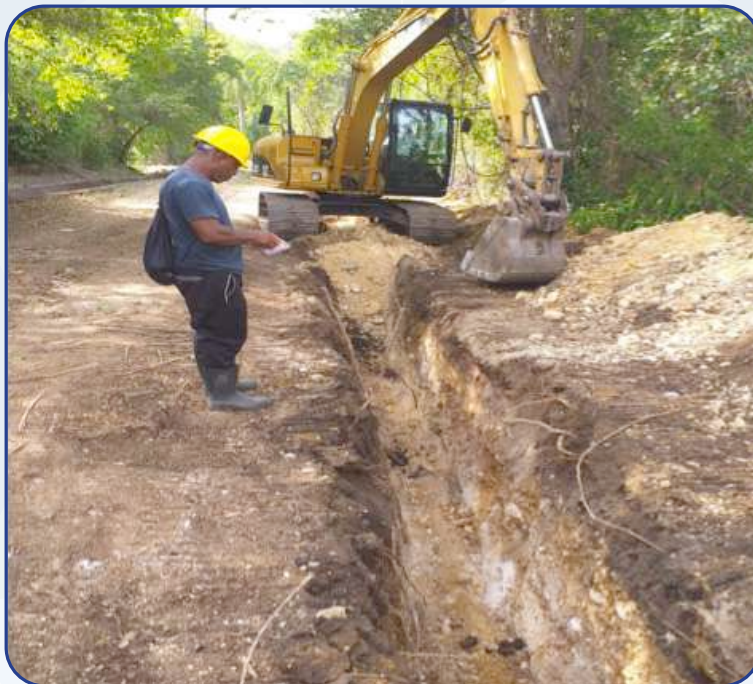
St. Jago North Spring Plain Extension work in progress
